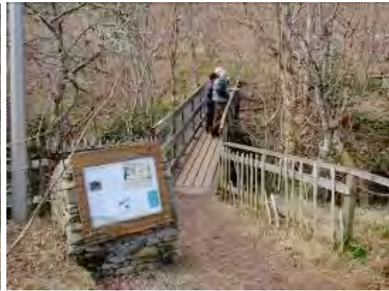
Fig. 3- View of footbridge from east
